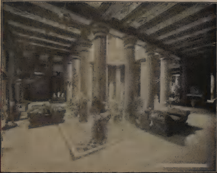
PERISTYLE OF THE POMPEIIAN HOUSE AT SARATOGA SPRINGS, N. Y. Franklin W. Smith, architect.
